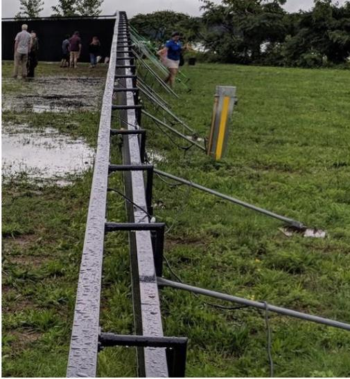
At the center point or apex of The Wall, the panels are slightly more than 7 ½ feet in height. Like The Wall, the panels slope from their apex height to 3-inches at the ends. The framework for these panels set on baseplates that are hammered into the ground using stakes approximately 18-inches in length.
